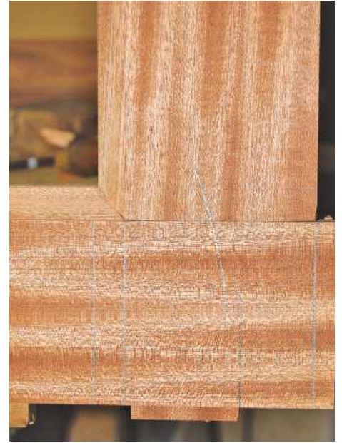
▲ Pic.17 One of the many mortise & tenons being fitted together
